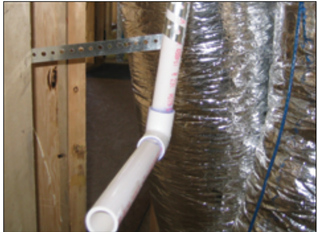
Figure 12-6 Sink Rough-In (Poor)
