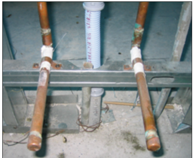
Figure 12-11 Appropriate Dissimilar Metal Isolation
