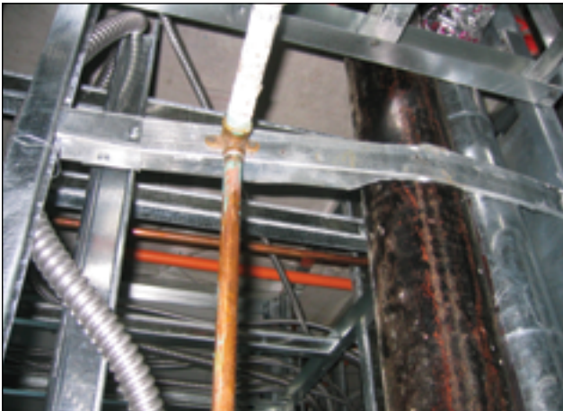
Figure 12-9 Showerhead Rough-In (Poor)
