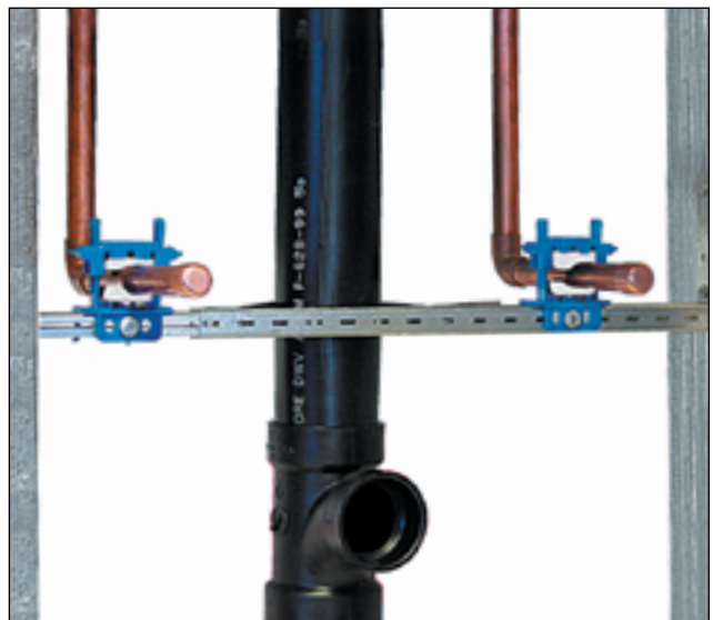
Figure 12-11 Appropriate Dissimilar Metal Isolation
