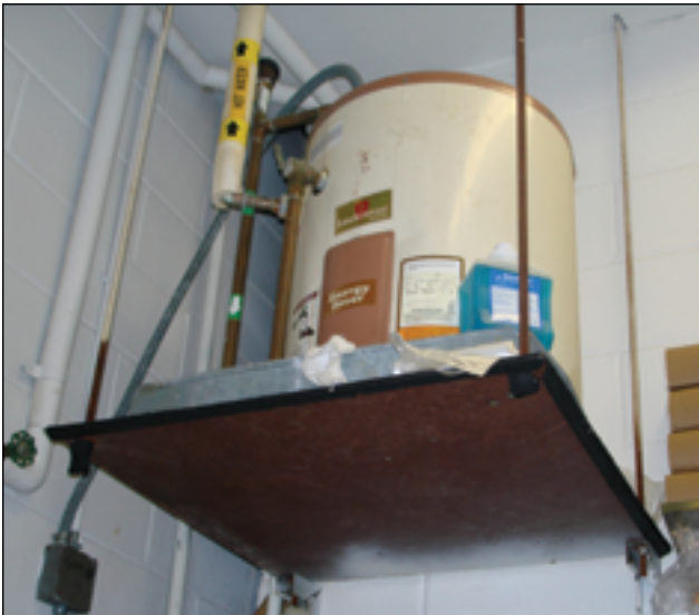
Figure 12-14 Makeshift Suspended Equipment Platform
