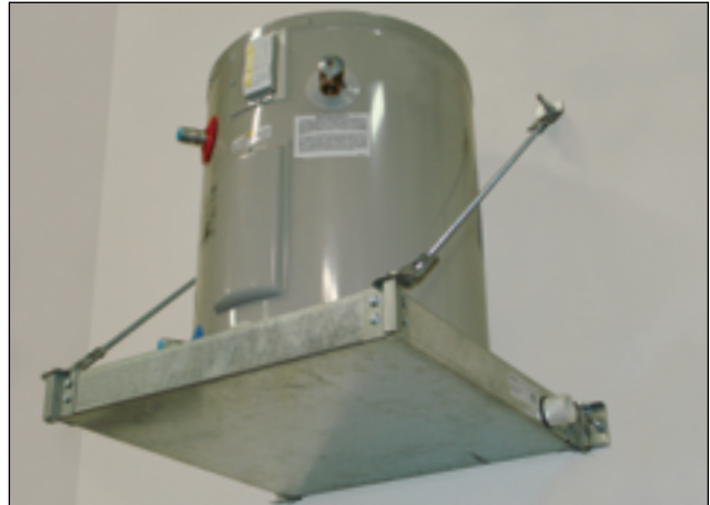
Figure 12-16 Engineered Wall-Hung Equipment Platform
