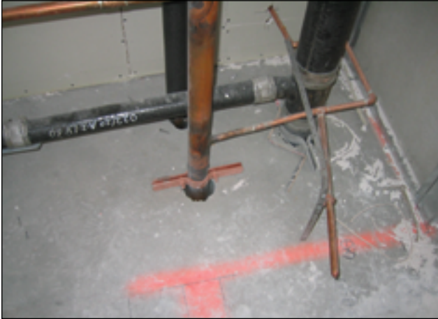
Figure 12-9 Showerhead Rough-In (Poor)
