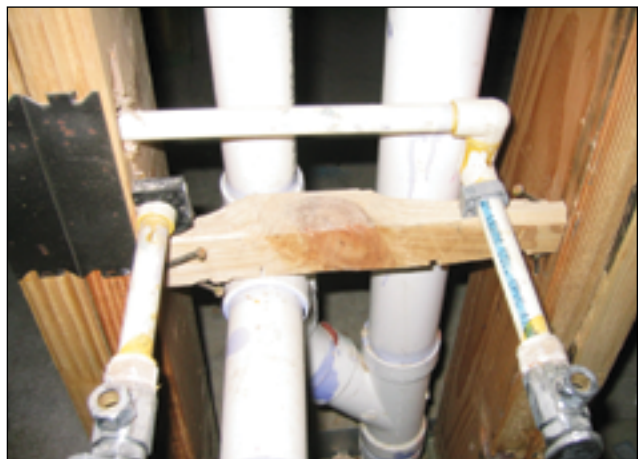
Figure 12-6 Sink Rough-In (Poor)
